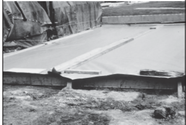
Slab on grade covered with waterproof paper for curing.
