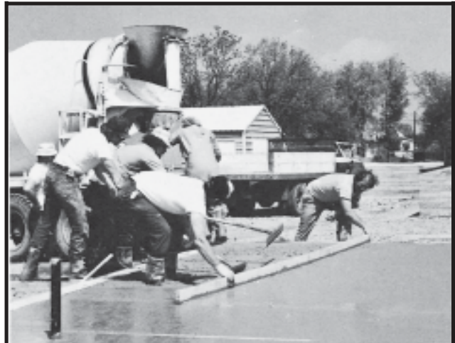
Finishing Concrete Flatwork
