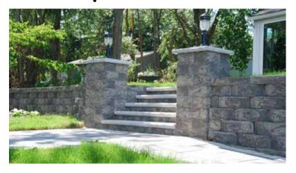
A gravity wall is a type of retaining wall that uses the force of gravity or the weight of the blocks that make up the wall to stand up and retain the area behind it. Most gravity walls use the principal of setback to make a stable wall without the use of reinforcement. Gravity walls tend to be shorter in height. There are options to build taller gravity walls, depending on the soil conditions and type of retaining wall system used.
